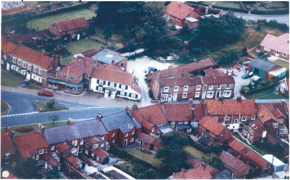
Aerial photo – 13 July 1974
