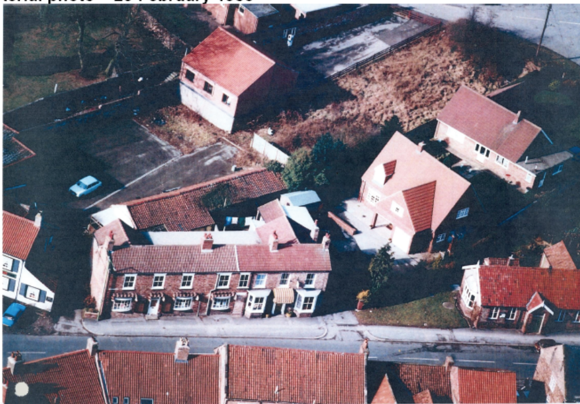
Aerial photo – 23 February 1985
